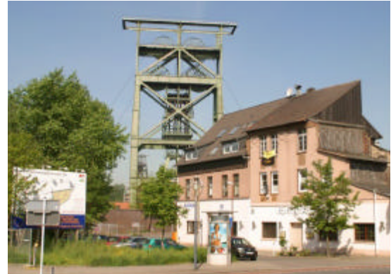
Abandoned Mine Site
